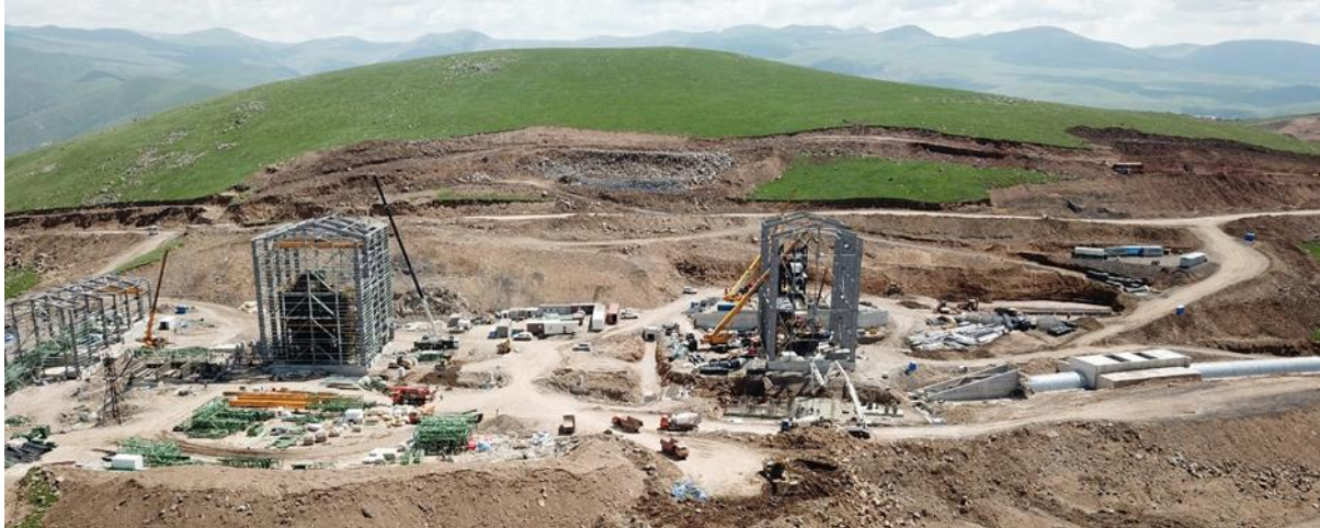
Figure 4-4: Construction at PL12 (Crusher)
