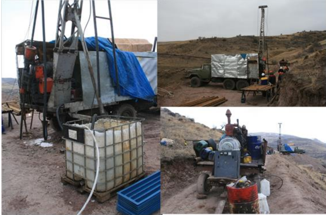
Figure 10-2: Drilling Operations Amulsar Project
